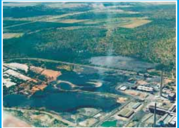
A typical lead slag dump
